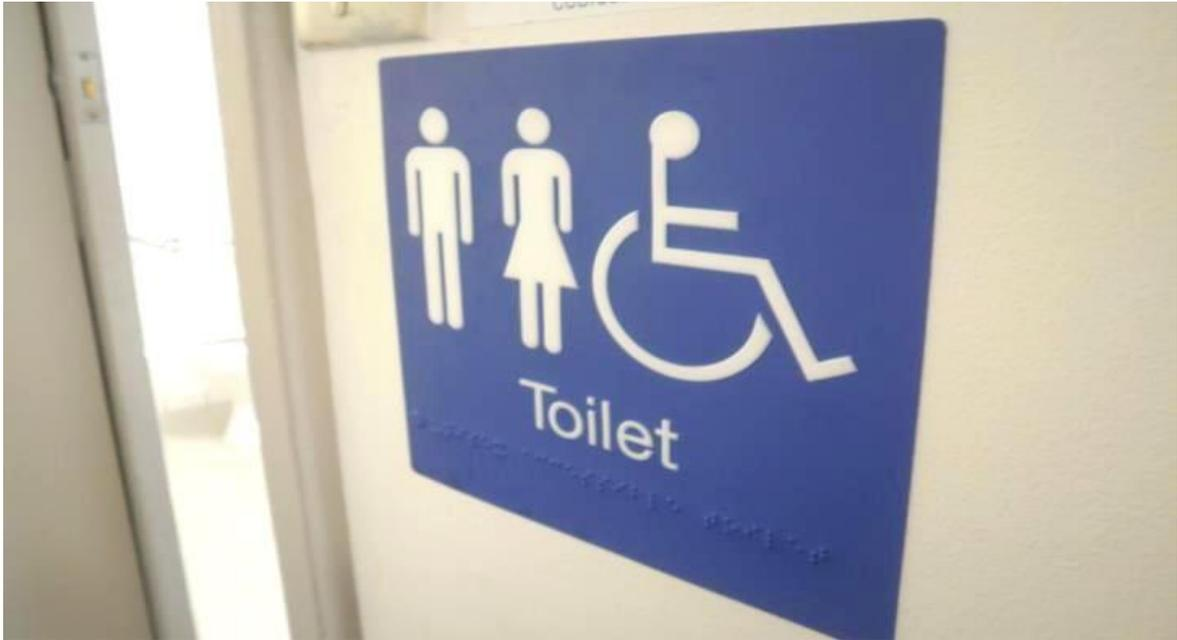
Fig.-11 Signage Panels with textual, braille and pictographic information with high colour contrast
